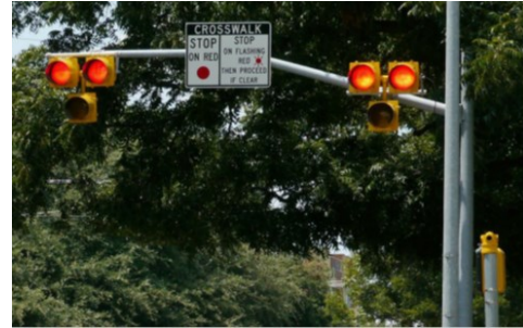
Pedestrian hybrid beacons, one of the safety countermeasures in the EDC-4 STEP program, alert drivers to the presence of pedestrians in a crosswalk.
